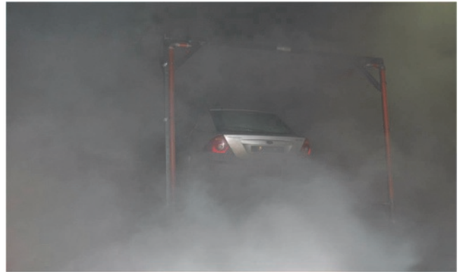
Sprinkler test terminated after 1 hour of sprinkler operation
